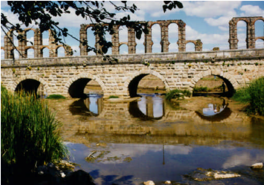
Fig. 3: Bridge over the Albarregas River in Mérida
