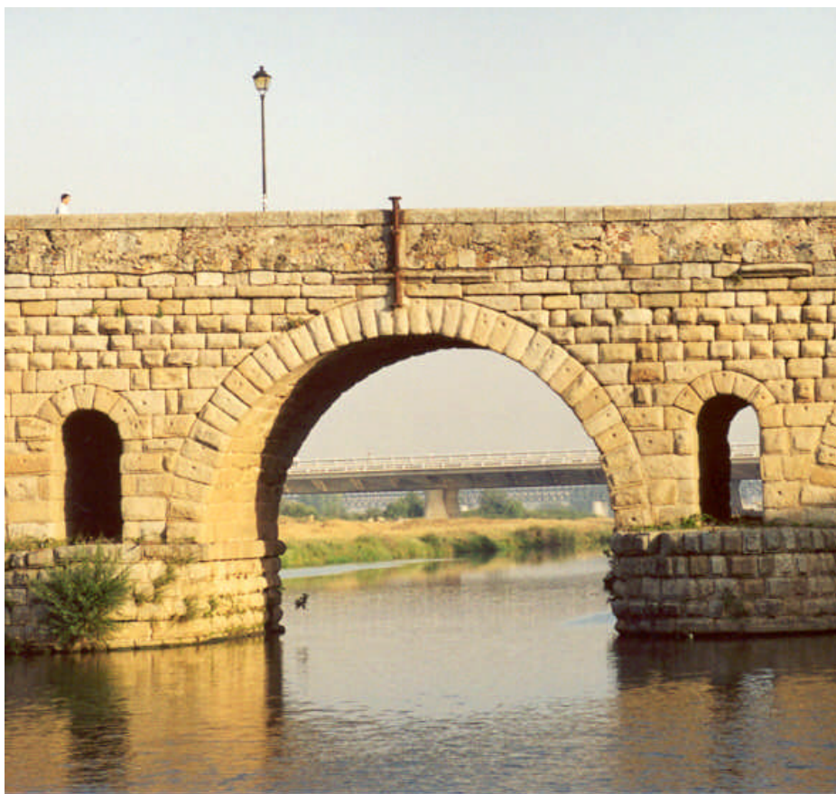
Fig. 4: Bridge over the Gadiana River in Mérida
